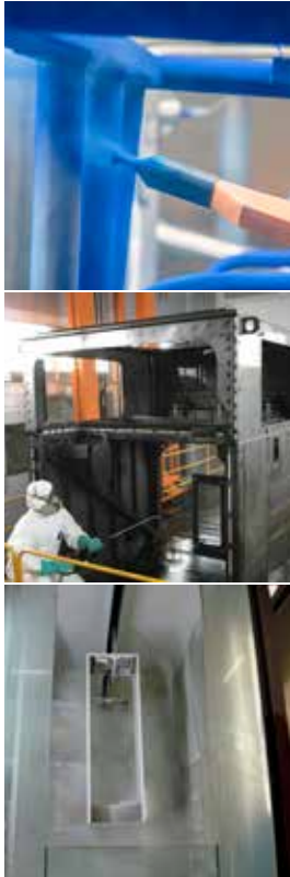
Image 1: Custom coater applying paint to production part after UniCoat® CTR application
